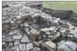
Side cell built into wall
