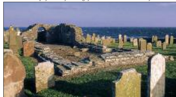
Cross Kirk at Tuquoy, Westray was largely demolished in the 18 th century
