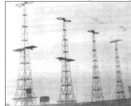
RAF Netherbutton transmitter pylons were 110m high
