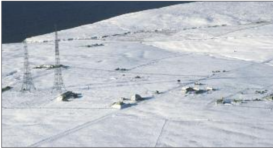
Netherbutton, Holm, the most northerly of the "Chain Home" radar sites
