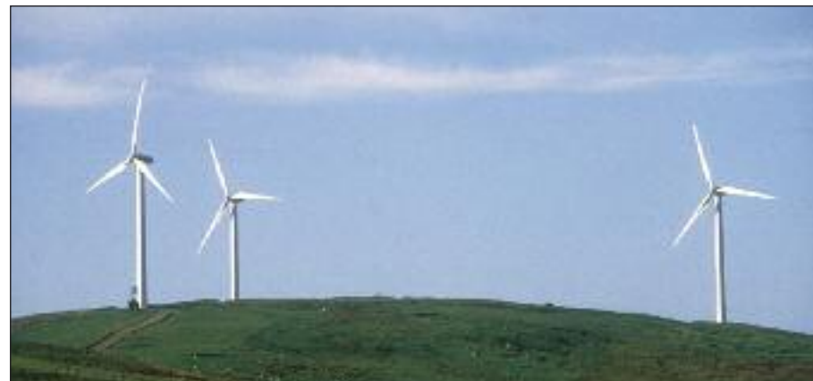
Burgar Hill Wind Turbines
