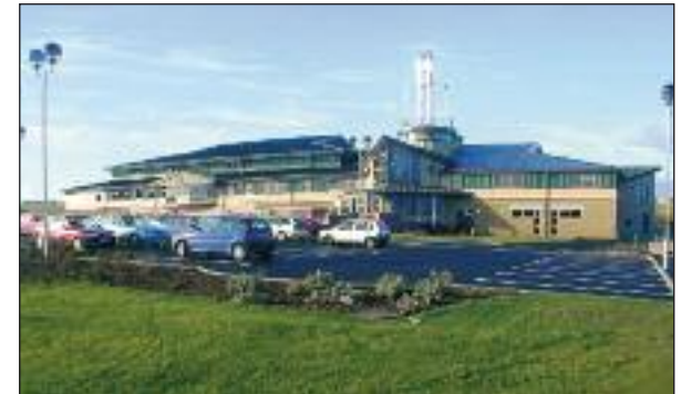
The Pickaquooy Centre offers many facilities, indoors and out
