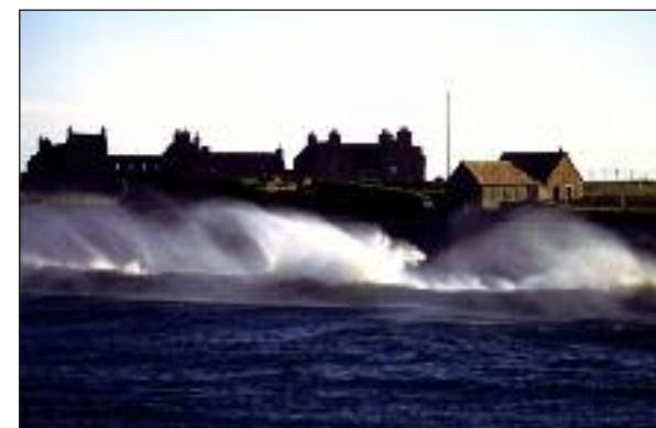
Waves breaking over the seawall onto Skara Brae
