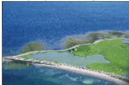
Aerial view of Damsay with its ruined buildings
