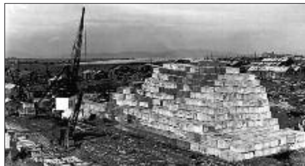
Over 50,000 concrete blocks were cast to clad the Barriers
