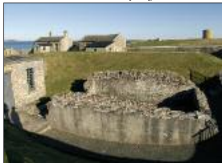
Hackness Gun Battery Magazine with blast-wall
