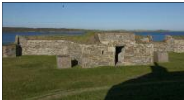
Martello Battery at Hackness showing embrasures and ready use magazine
