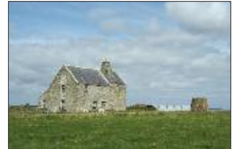
The New Mill at Nesstoun and the stump of a windmill
