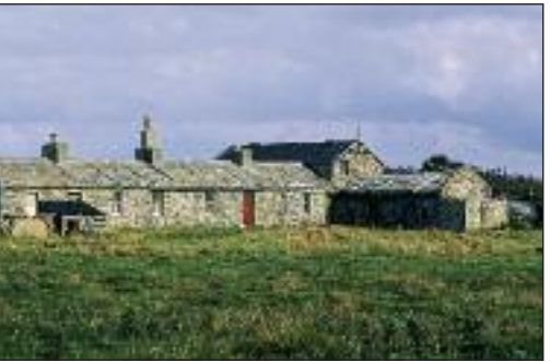
Typical North Ronaldsay croft with a flagstone roof
