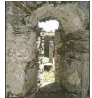
Window interior view
