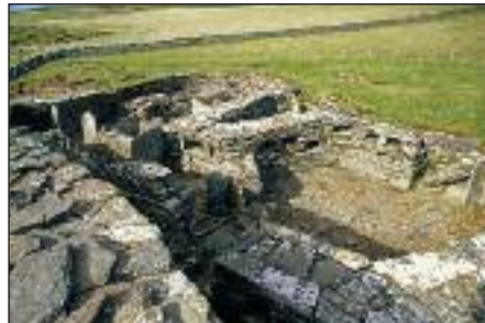
Ruinous buildings on the outside of the broch tower
