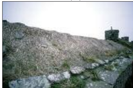
Ortie, Burness - detail of roof construction with simmons
