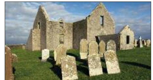
Old Lady Kirk is now roofless and was built or renovated in 1773
