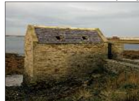
Sea-washed toilet at the west side of the village
