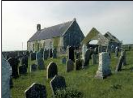
The "Old Kirk" is now roofless
