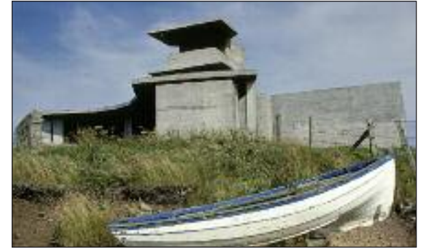
Galtness WWII Coastal Battery house a twin 6-pounder gun
