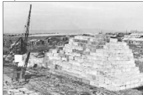
Blocks for the Churchill Barriers
