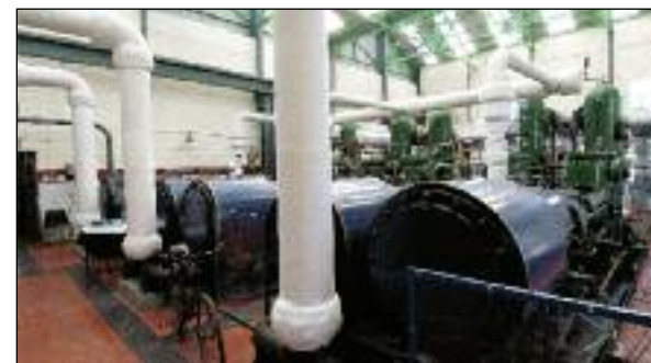
Scapa Flow Visitor Centre Pump House
