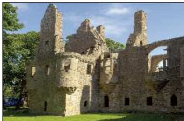
The Earl's Palace was built about 1600
