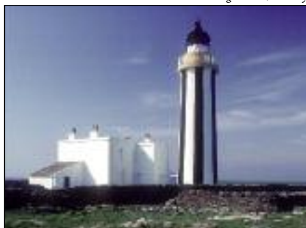
Start Point lighthouse, Sanday
