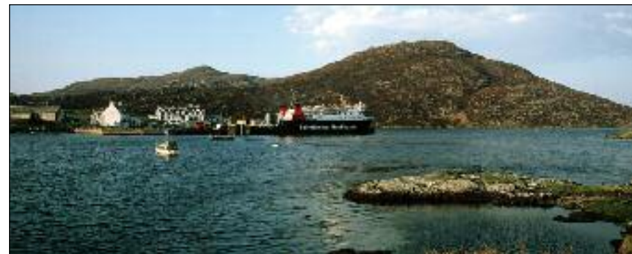
Lochboisdale from the south with Beinn Ruigh Choimnich (280m) in the background
